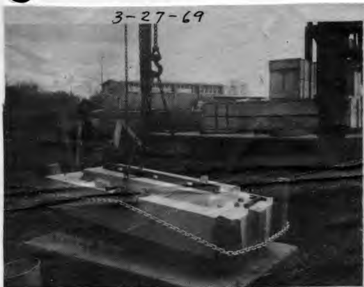
Here workmen place the base of Wheeling's Veterans Memorial on a foundation of seven square yards of solid concrete, the start of the five sections needed for completion.
