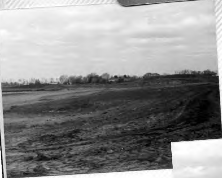
Heritage Park Retention Basin Nicknamed "Yecca Flats"
