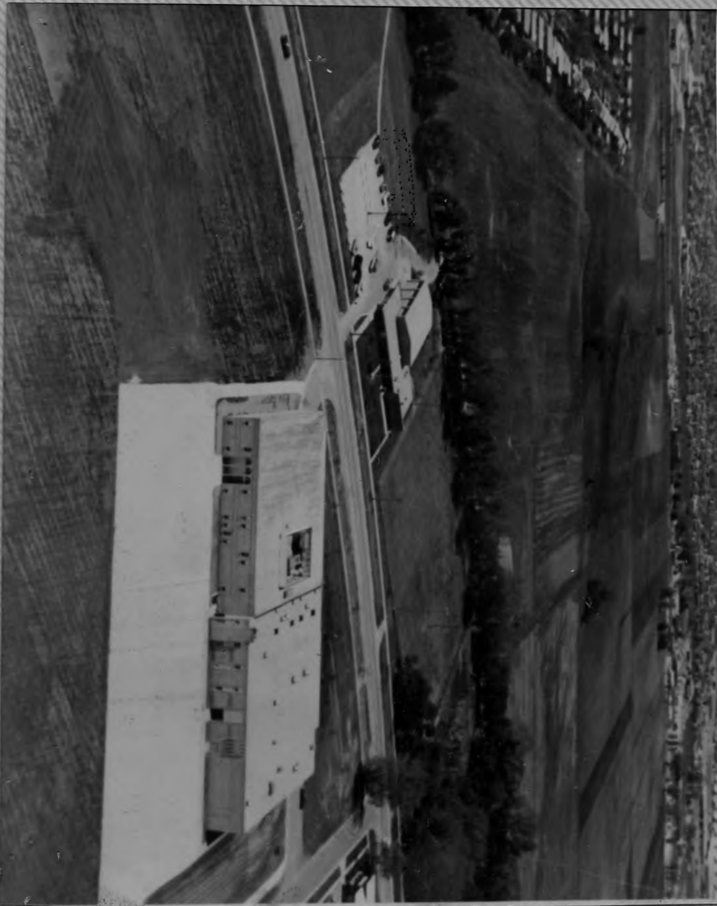
HERITAGE PARK - HOLMES SCHOOL AIR VIEW
